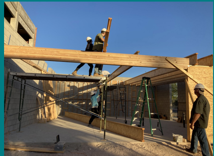
Students constructing Rowhouse 4
