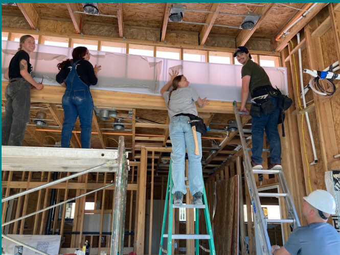
Students constructing Rowhouse 3
