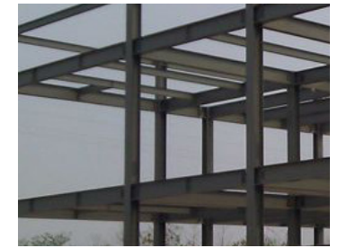
DARK GRAY STRUCTURAL STEEL FRAME
